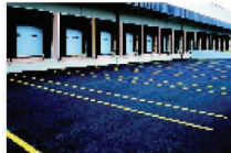
Rampa Sistemli Kapılar / Doors with ramp systems
